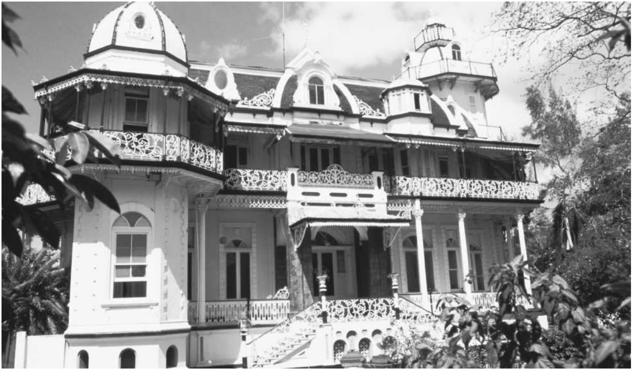
Iron lacing decorates a colonial style mansion in Port of Spain, Trinidad and Tobago.
